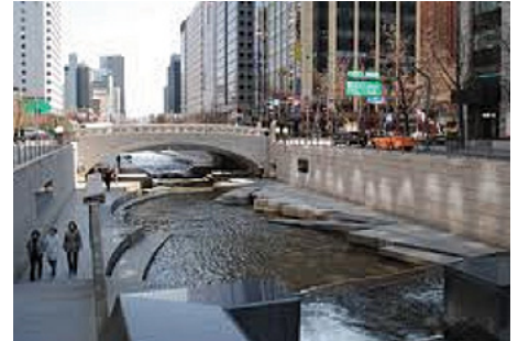
Bridge crossover the stream
