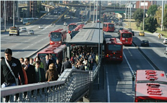
Busway and traffic lanes accessed by the pedestrian bridge
